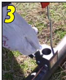
3 Place metal disc in bottom of mold.
