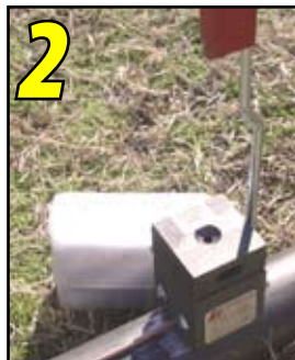
2 Position conductor and mold onto pipe.
