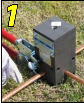
Position cleaned conductors in mold
