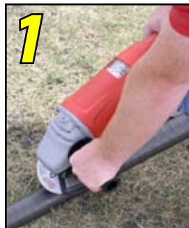
1 Clean pipe before making weld.
